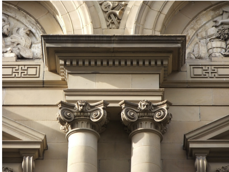
Figure 11. An example of segment of entablature, a continuous horizontal lintel that is supported by columns; applied in the Parthenon and Pantheon as previously discussed. From Image Ionic capitals and entablature, Free Trade Hall, Manchester, by Orangeaurochs, 2011, https://www.flickr.com/photos/orangeaurochs/5763101886 . © 2011 by Orangeaurochs.
