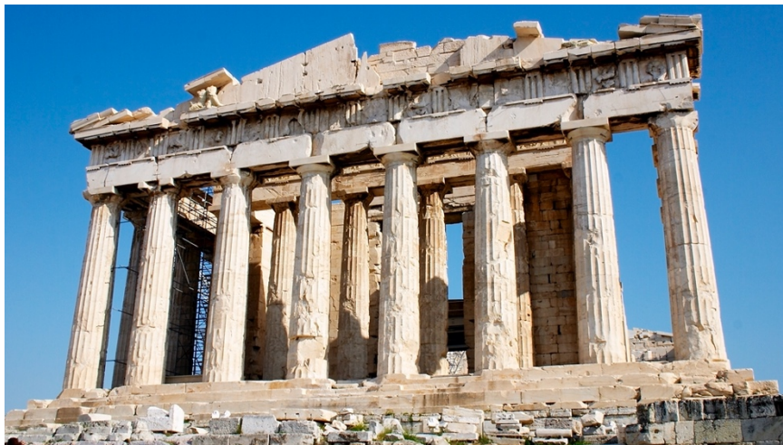
Figure 12. An example of colonnade, a row of columns that support a roof, as demonstrated in this picture of the Parthenon. Their purpose is both structural and aesthetic. From Image Parthenon-Restoration-Nov-2005-a, by Barcex, 2005 https://commons.wikimedia.org/wiki/File%3AParthenon-Restoration-Nov-2005-a.jpg . © 2005 by Barcex.
